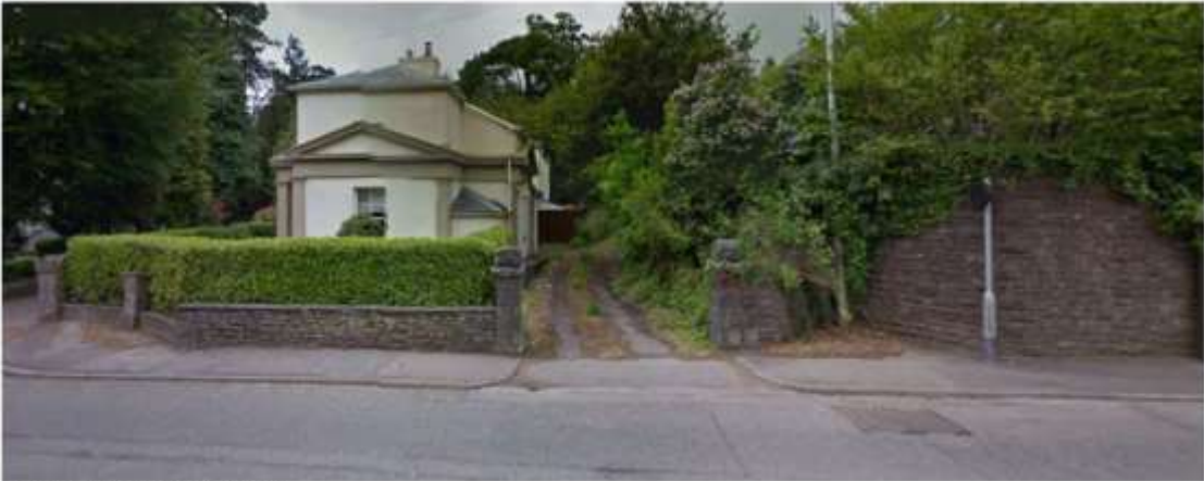
Existing access from the A48
